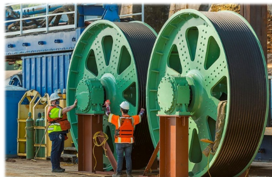
I-5 Bridge Trunnion Project
