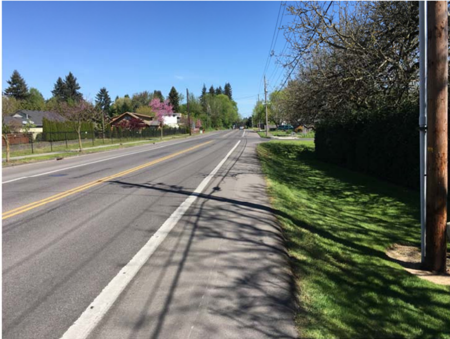
Rough, uneven terrain forces pedestrians onto the roadway.
