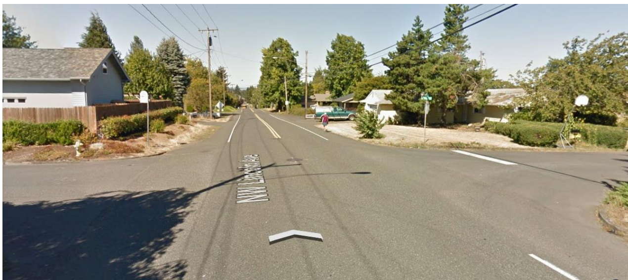
Lincoln and NW 49 th Street Looking North – Sidewalks on the west side of Lincoln would prevent pedestrians from having to use the unprotected shoulder; the bus stop at the northwest corner of intersection would become accessible for all users; the proposed RRFB at this intersection would create a safe crossing for all users and provide safe access to the proposed pedestrian path shown below.
