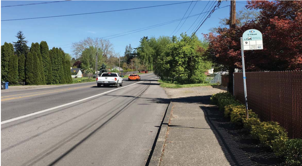
Intermittent sidewalk ends abruptly.
