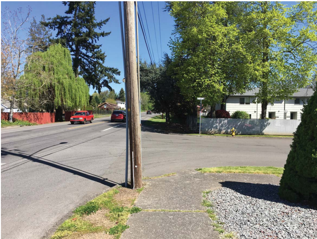
Intermittent sidewalk ends and curb ramps non-compliant/missing.
