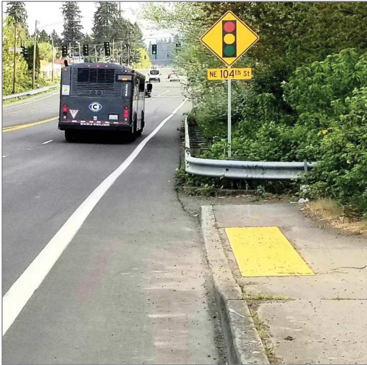
End of sidewalk Hwy 99 near NE 102nd Street – Looking north
