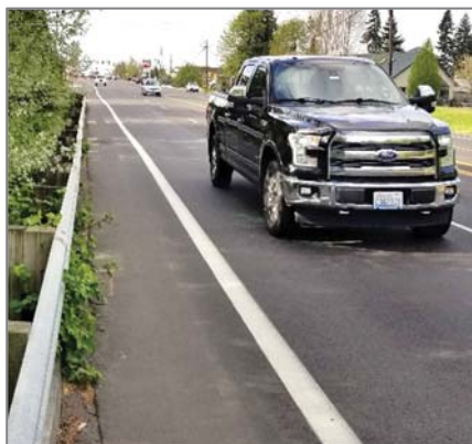
Ped/Vehicle Conflict Hwy 99
