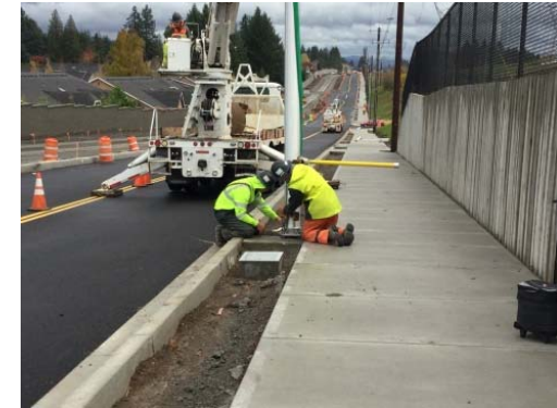
Vancouver: NE 18 th Street Construction
