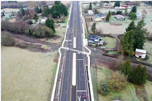
NE 119 th Street RR Crossing
