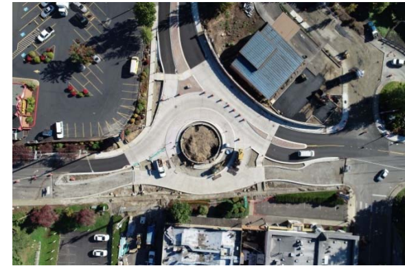
La Center: 4th Street & Pacific Hwy Roundabout
