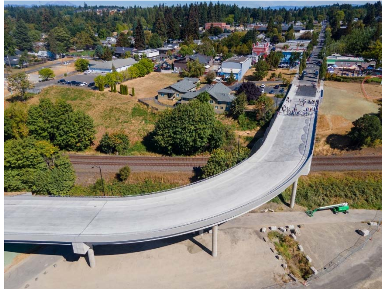
Port of Ridgefield: Pioneer Street Railroad Overpass
