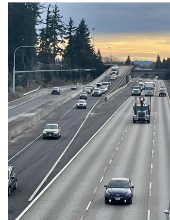
I-205/Mill Plain NB Ramp Meter
