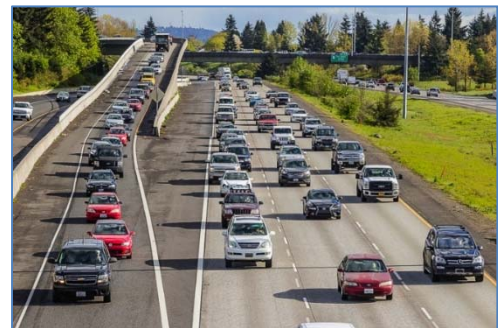
I-205 at Mill Plain Ramp Meter
