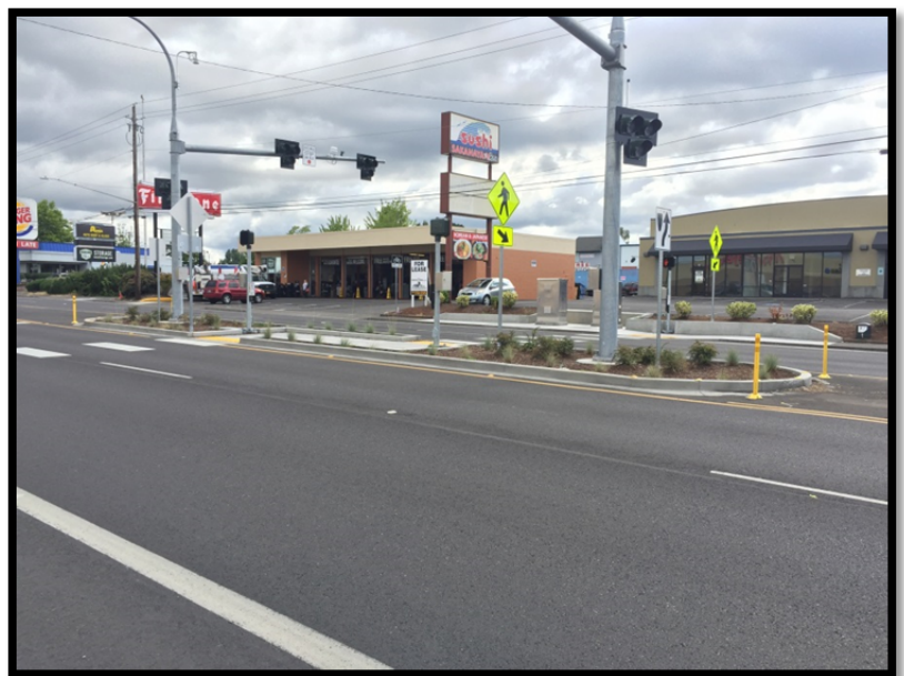
After construction – HAWK
