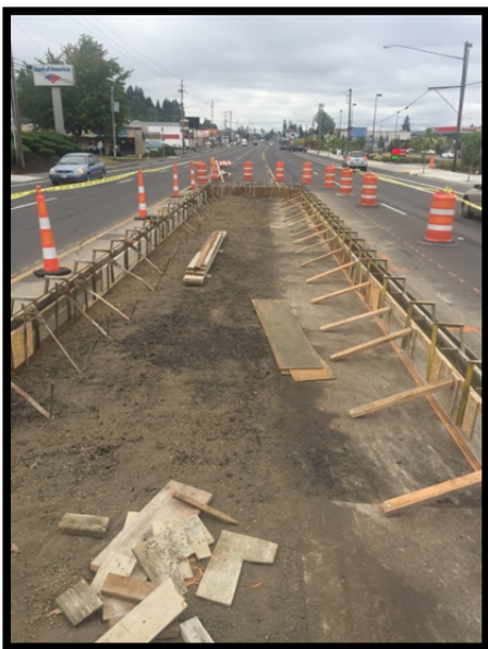
During construction – HAWK
