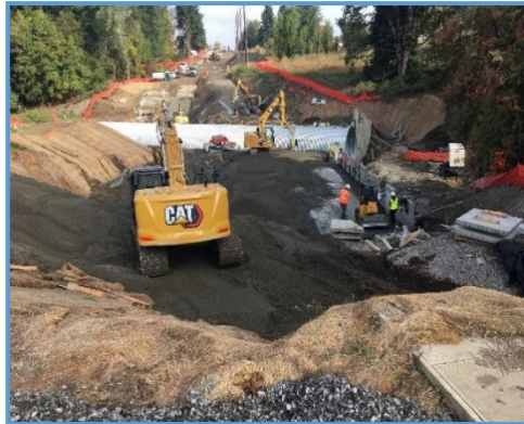
Construction NE 10th Avenue near NE 148 th Street Looking North
