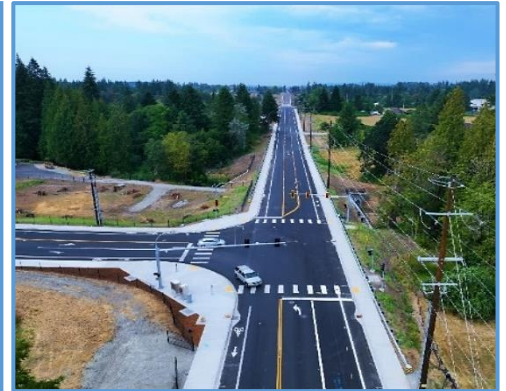
After NE 10th Avenue near NE 148 th Street Looking North
