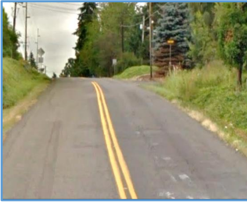
Before NE 10th Avenue at NE 149 th Street Looking South
