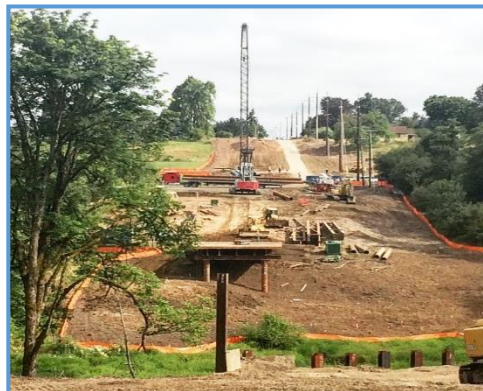
Construction NE 10th Avenue at Whipple Creek Looking North
