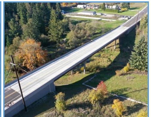
After NE 10th Avenue at Whipple Creek Looking North
