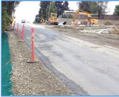
Construction NE 10th Avenue at NE 149 th Street Looking South
