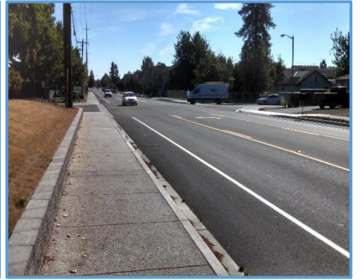
After NE 10th Avenue at NE 149 th Street Looking South
