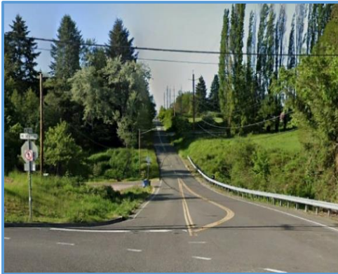
Before NE 10th Avenue near NE 148 th Street Looking North
