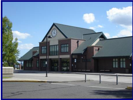
Fisher's Landing Transit Center
