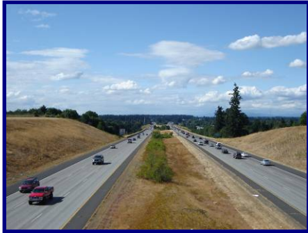
I-205 near Burton Road
