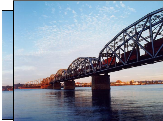
RN BNSF Columbia River Bridge with open swing span
