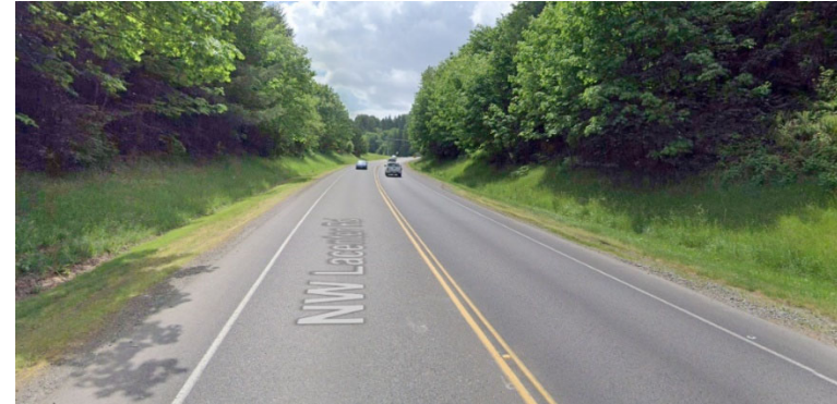
Figure 6. Street view traveling southwest on La Center Road
