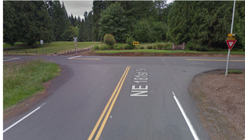
Figure 7. NE 181st Avenue Northbound Approach to NE 152 nd Avenue
