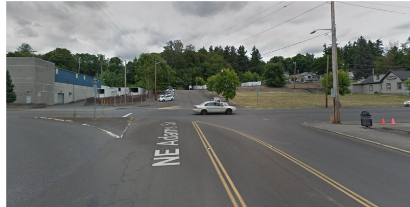
Figure 9. NE Adams Street Northbound Approach at NE 6th Avenue
