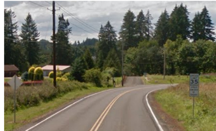
Figure 7. NW Pacific Highway, westbound horizontal curve with visual trap
