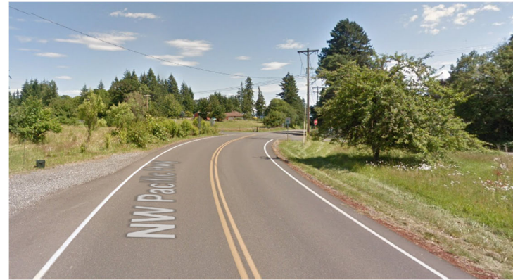
Figure 12. Horizontal curve approaching the intersection
