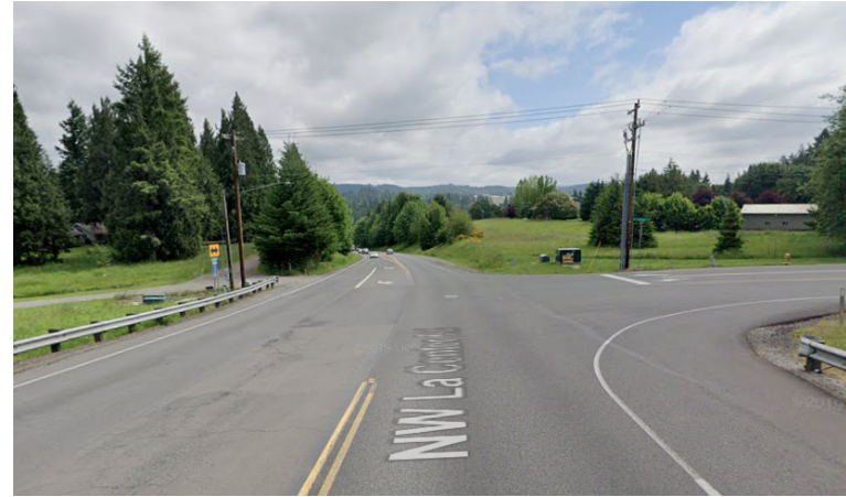
Figure 13. Eastbound La Center Road at Timmen Road
