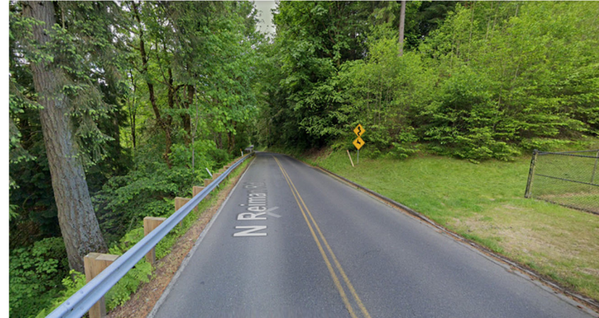
Approaching Horizontal Curve on N Reiman Rd/NW 51st Ave
