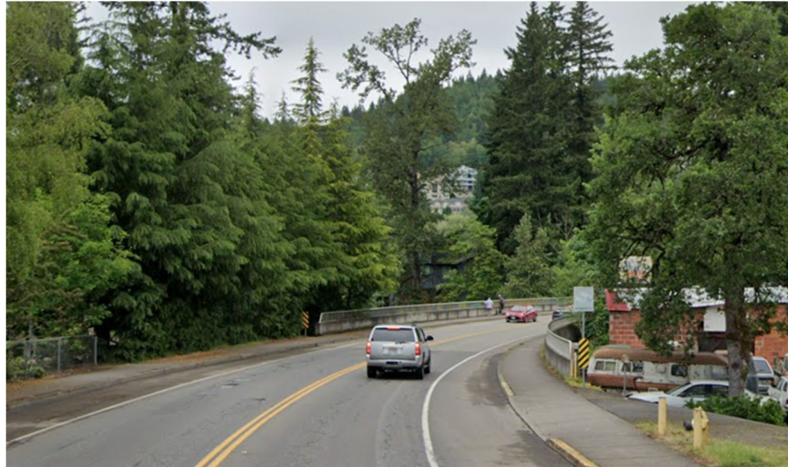
Figure 9. Facing northbound on Washougal River Road and approaching bridge crossing.
